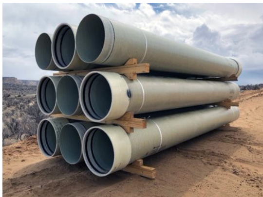
Fiber-reinforced polymer (FRP) pipe ready to be installed at a Reclamation project.
